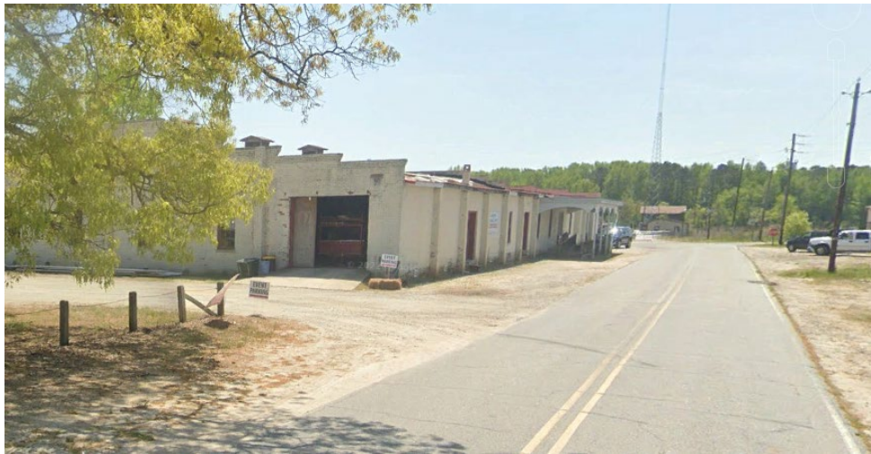
Figure 4-11. Existing Conditions along Barnes Street
